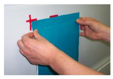
For proper positioning put reference marks onto the substrate. Use masking tape or any other easy to remove marker.
