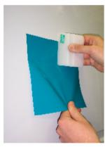
Start application at the middle of the already applied edge. Use a squeegee and firm pressure and apply marking in overlapping strokes from the center to the edges. Work towards your other hand still holding the marking off the substrate.
