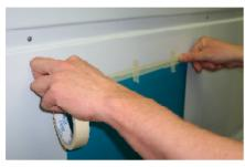
Create a horizontal tape hinge at the top of the marking.
