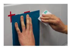
Bubbles can be pricked with a needle and squeezed out.
