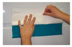
Turn over marking and remove and fold ca. 20 cm. of the liner.
