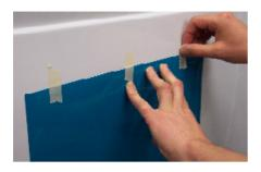
Position liner and marking on substrate using masking tape.
