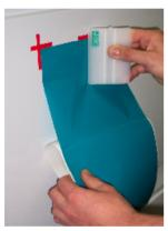
Remove ca. 20 cm. of the liner. Keep marking close to substrate without contact. Start application at the middle of the already applied edge. Use a squeegee and firm pressure and apply marking in overlapping strokes from the center to the edges. Work towards your other hand still holding the marking off the substrate. Repeat until liner has been removed completely.
